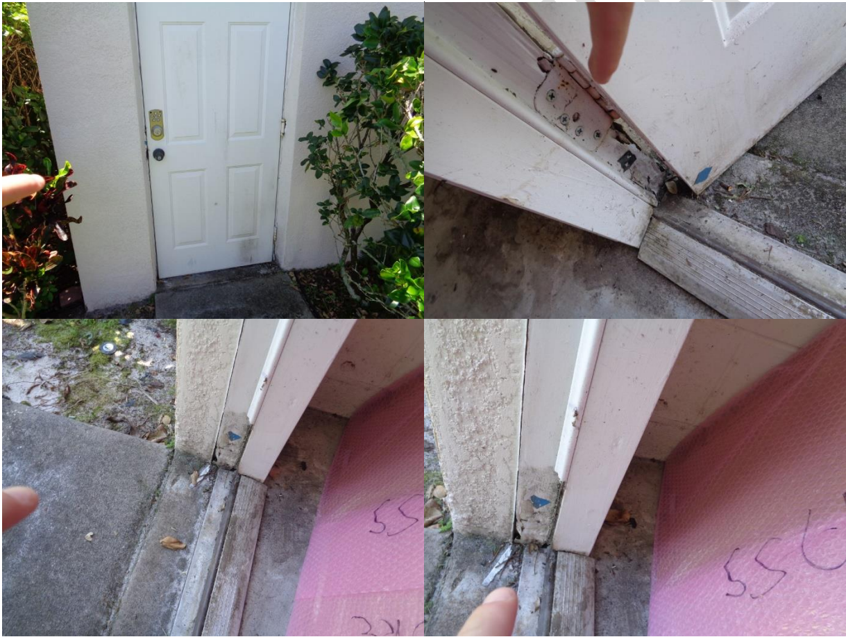
Damage trim and wood present around exterior personal garage door should be evaluated and repaired by a certified contractor.
