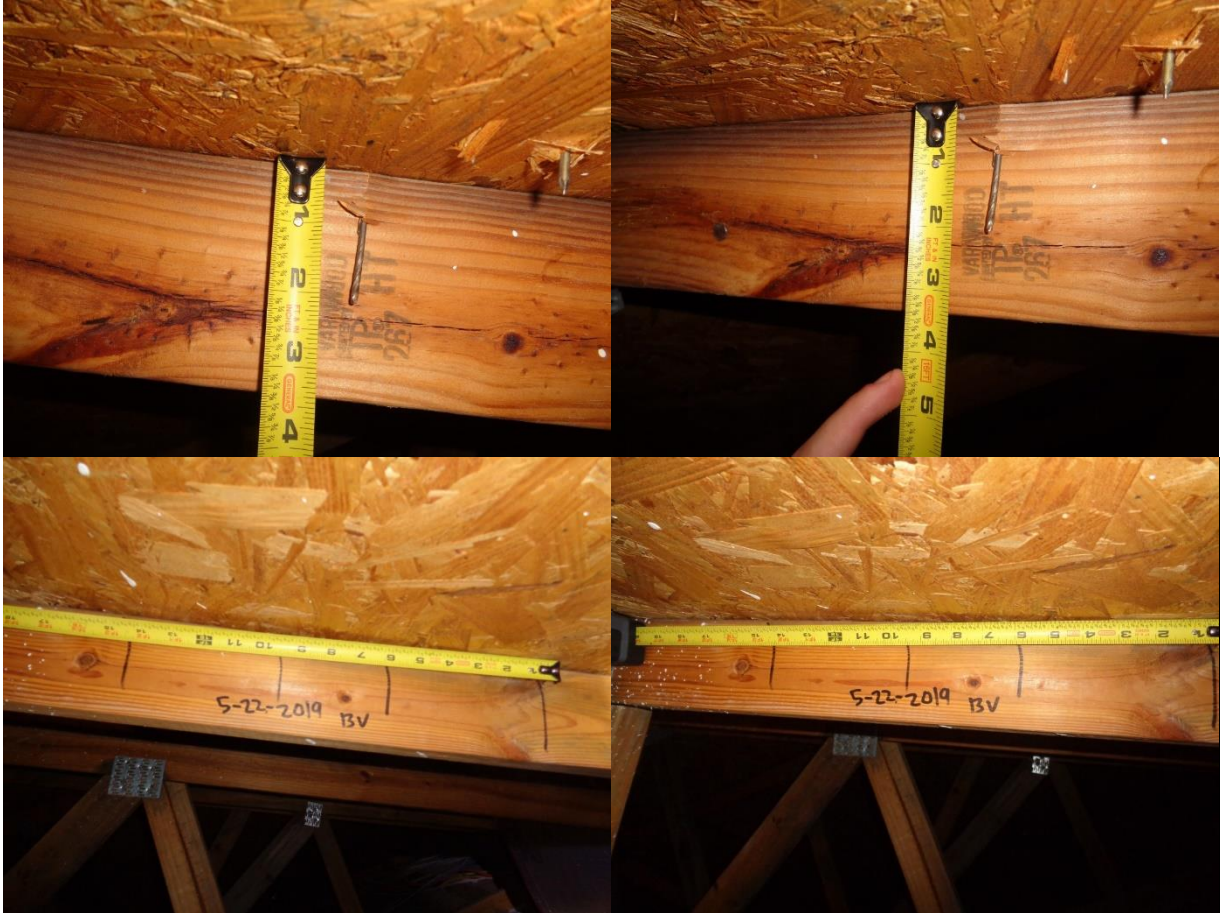
Roof Decking Attachment Nail Size & Spacing
