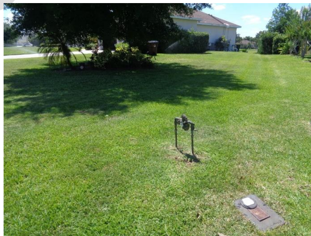
Backflow prevention value Location
