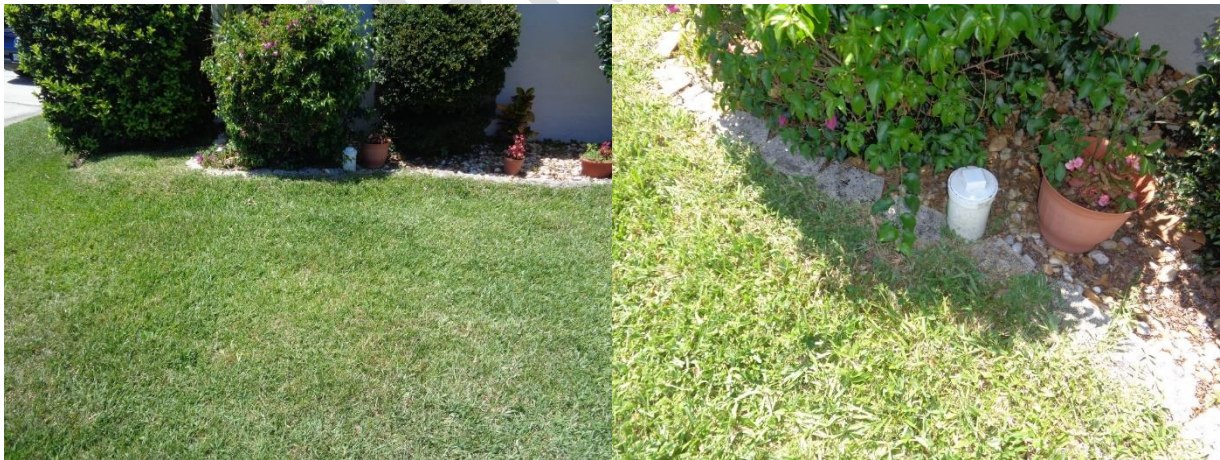
Private Septic Cleanout Location
