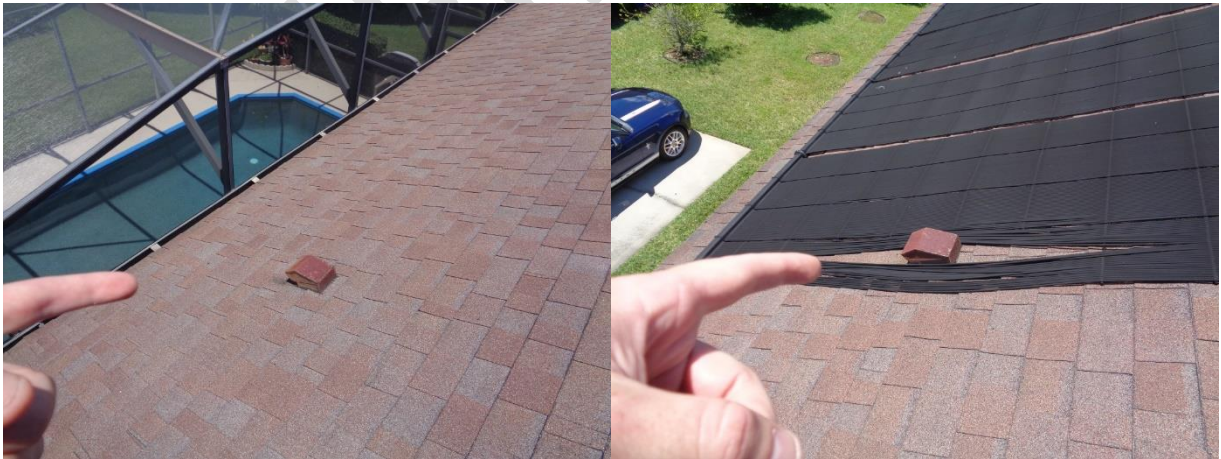
Exhaust vents had evidence of rust at time of inspection and should be repaired.
