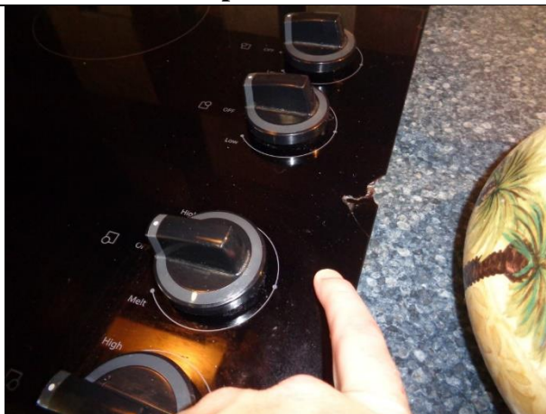
Damage to the stove top present at time of inspection and should be repaired
