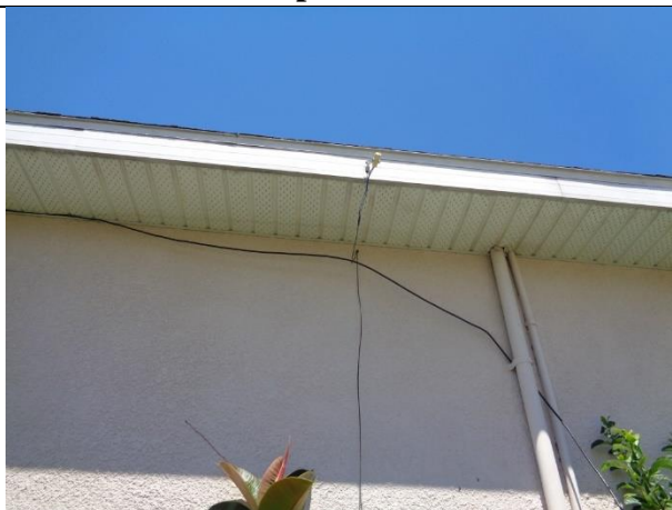
Rain Sensor Location
