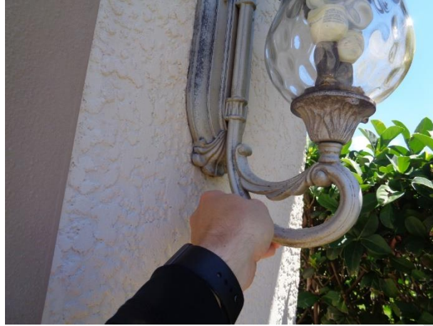
Front exterior wall mounted light fixtures were loose at time of inspections and should be secured and sealed.
