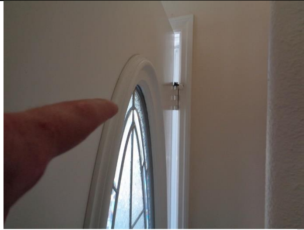
Door stopper did not operate correctly at the front door at time of inspection and should be repaired
