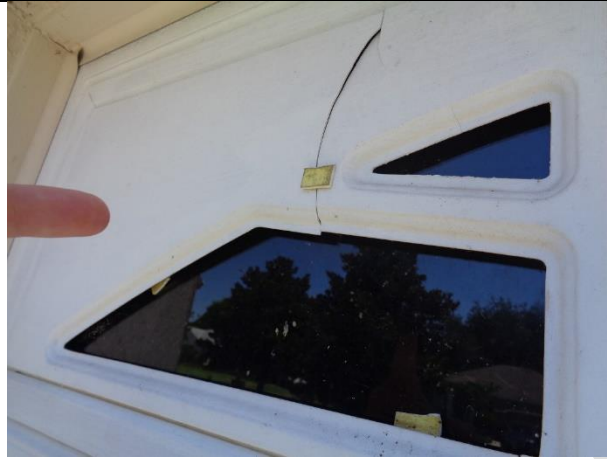
Damage to garage door window frame present at time of inspection and should be repaired
