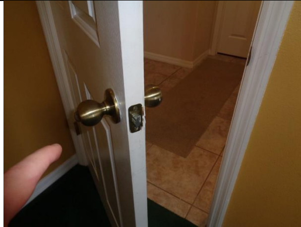
Locking mechanism for the door handle in the west bedroom did not lock at time of inspection and should be repaired
