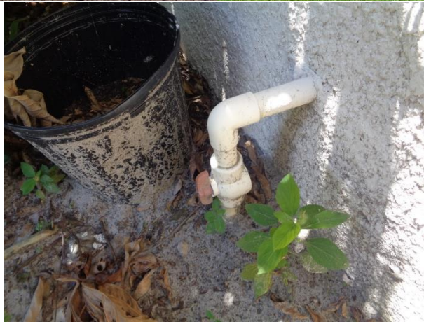
Water Meter Location - Main Shut off Valve Location
