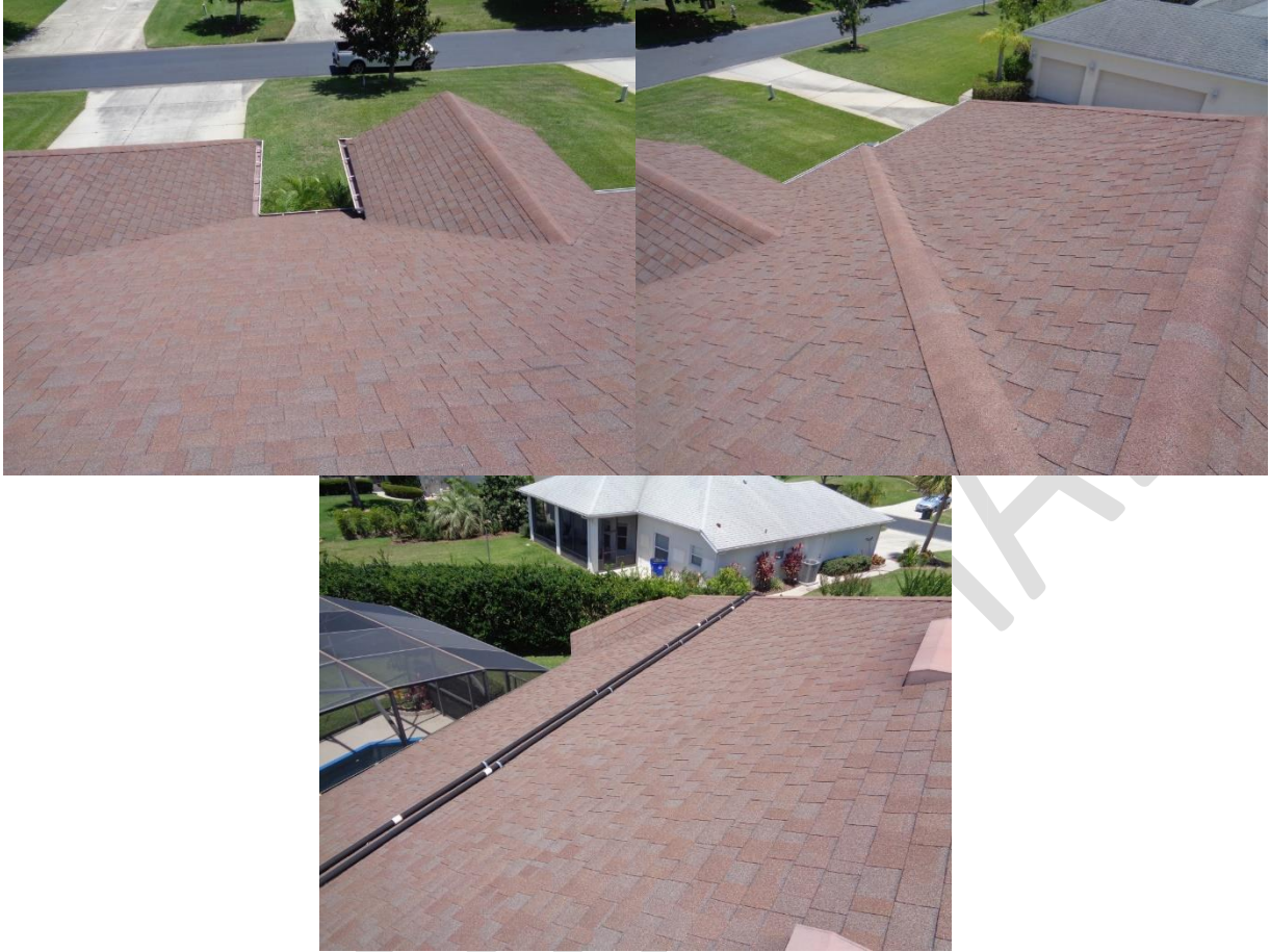
Type of roof covering
