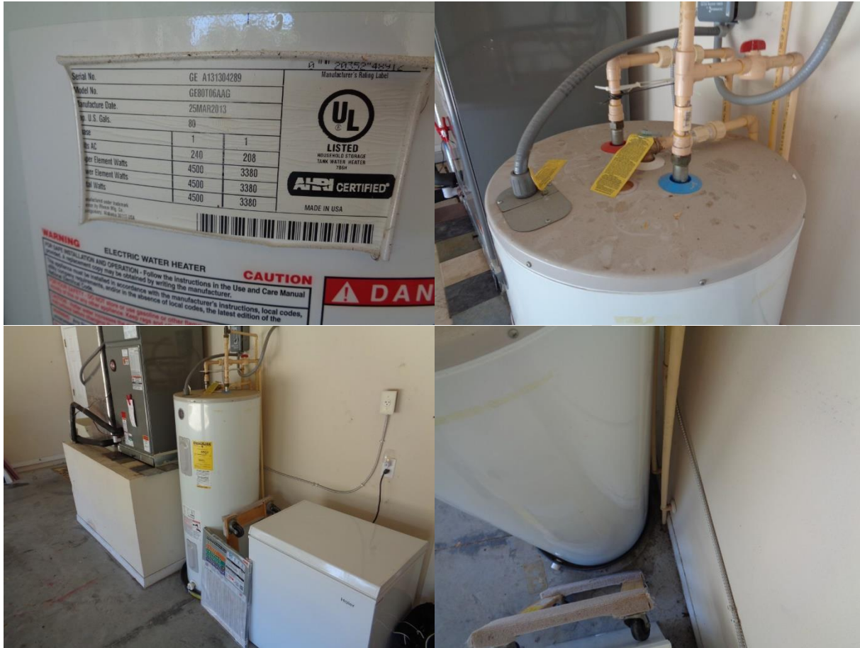
Water Heater Fuel Type - Water Heater Manufacturer - Water Heater Size
