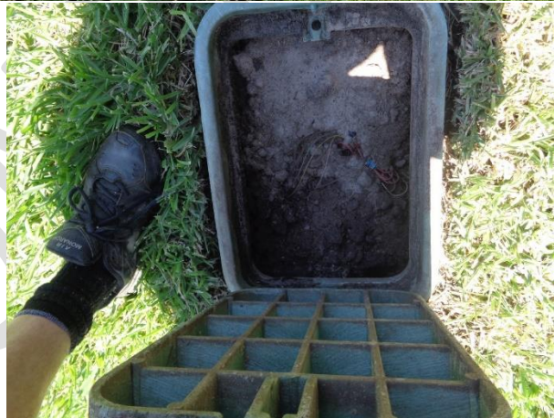
Irrigation valves location:
