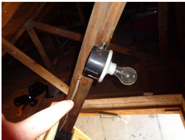
Install Light Bulb for the garage Attic Access Area Light Fixture
